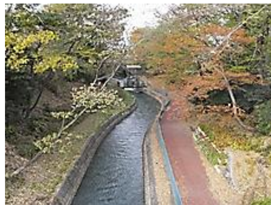
Fig. 1 Tenguiwa Irrigation Canal
